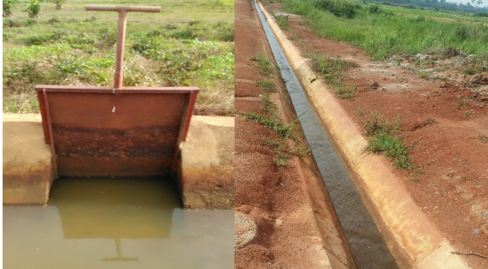
Figure 6 : Mobile gate repaired and main channel cleaned and rehabilitated
